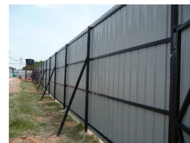
Hoarding Erected along Construction Site
